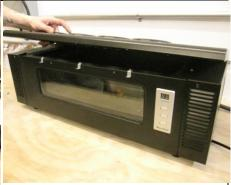
Install (3) Z-clips on front side only, securing each with a screw.
